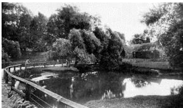
Former Mill in Kingsthorpe (site located to the south of the Conservation Area)
