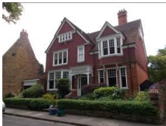
The Old Rectory on The Green, built of brick with tile hanging at first floor level
