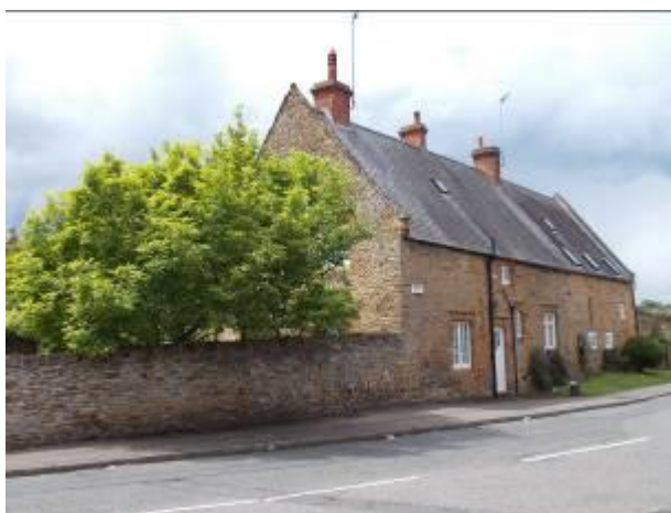
Home Farm House, dating from the 17 th century; the boundary wall forms the southern boundary of the Conservation Area.
