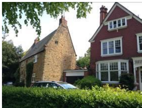
Buildings constructed in local sandstone, red brick and tiles in juxta position, built over separate centuries, is an attractive feature of the variety within the Conservation Area.
